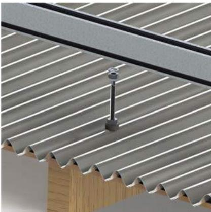
4. Place the second bolt and lower it to the planned rail height above the roof.
