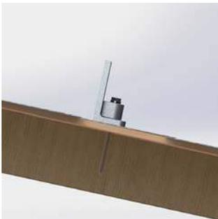
5. Screw the 5/16" lag bolt into the rafter, embedded a minimum 2.5". Tightening torque is dependent on the roofing material.
