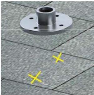
1. Drill two pilot holes using 3/16" drill bit through the roof material and into the center of the rafter at the planned location.
