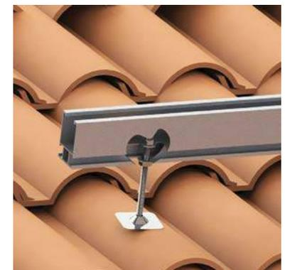
9. Attach the rail to the headless threaded bolt using two 3/8" nuts.
