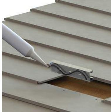
2. & 3. Insert the lag bolt through the tile strut and apply compatible sealant.
