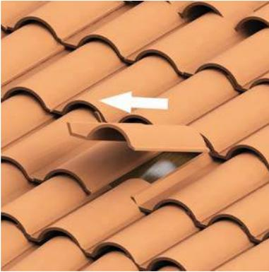
1. Remove the tile and locate the rafter.
